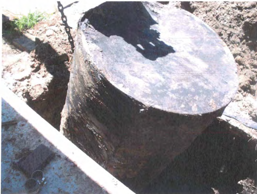
Picture 2: UST 130Banyan-1 during removal.
